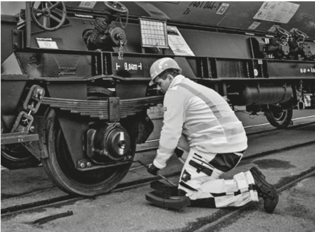
Mobile maintenance: replacing brake blocks
