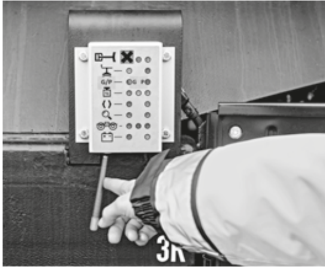
Key sensor data on the status of the braking system is displayed directly on the wagon for railway personnel.
